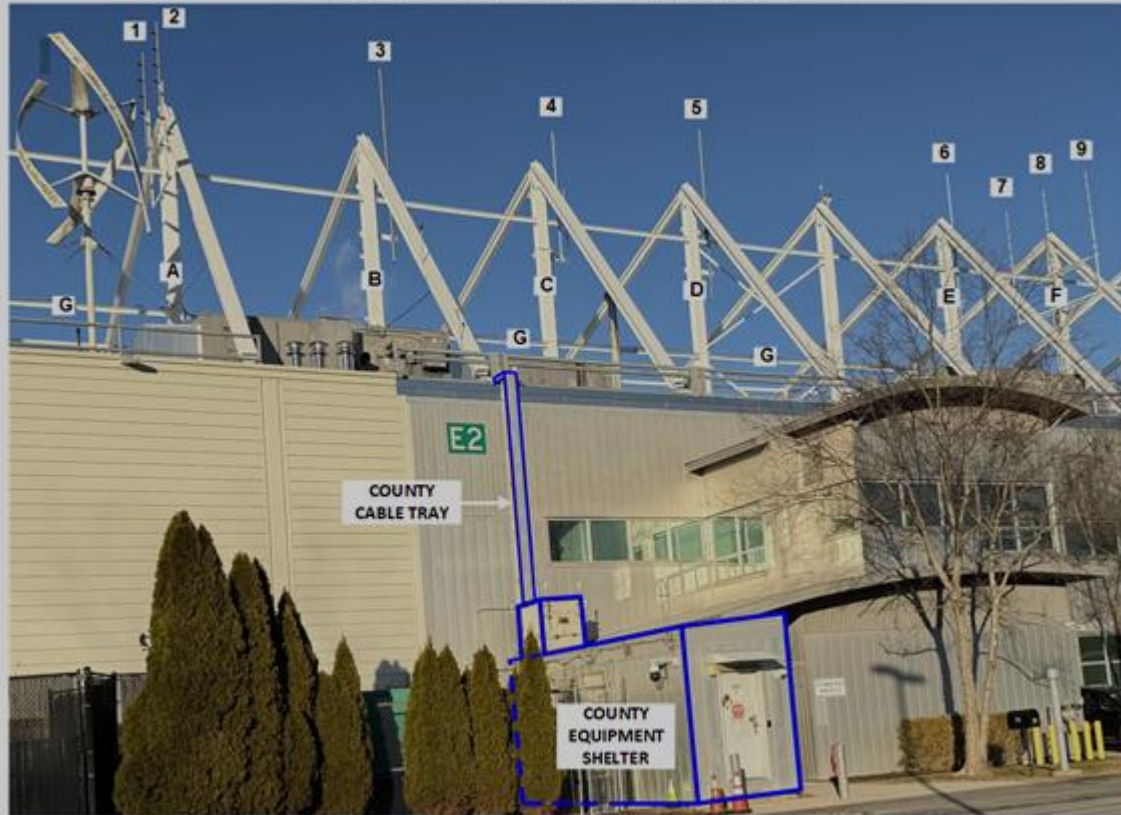
County Antenna Masts are numbered "1" through "9". County transmission lines to be routed inside County Cable Tray from County Equipment Shelter to steel column "C" on roof, clamped along lateral steel bracing "G" to steel columns "A", "B", "D", "E", and "F", and up steel columns "A" through "F" to County Antenna Masts "1" through "9". Existing County Antenna types are described on the following pages.
